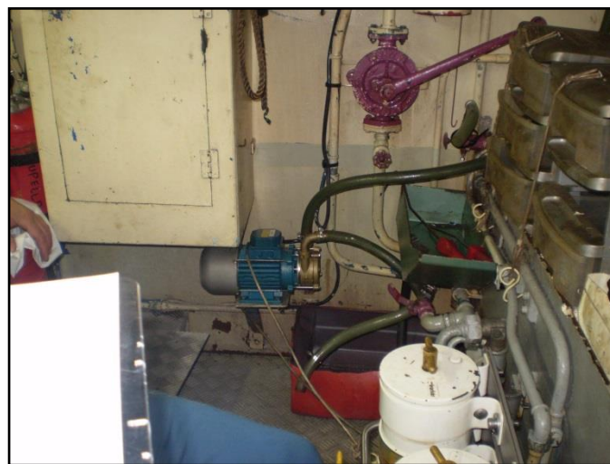
Pompe de transfert gasoil
