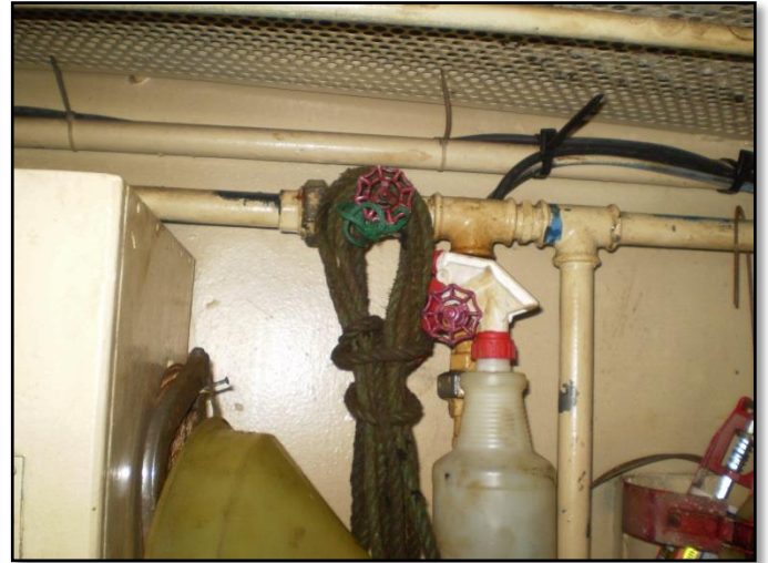
Vanne retour caisse gasoil Td
