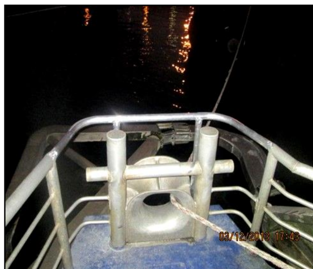
Altered safety rail
