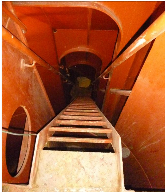
Figure 6: Internal view of the 'Australian ladder' showing the bottom
